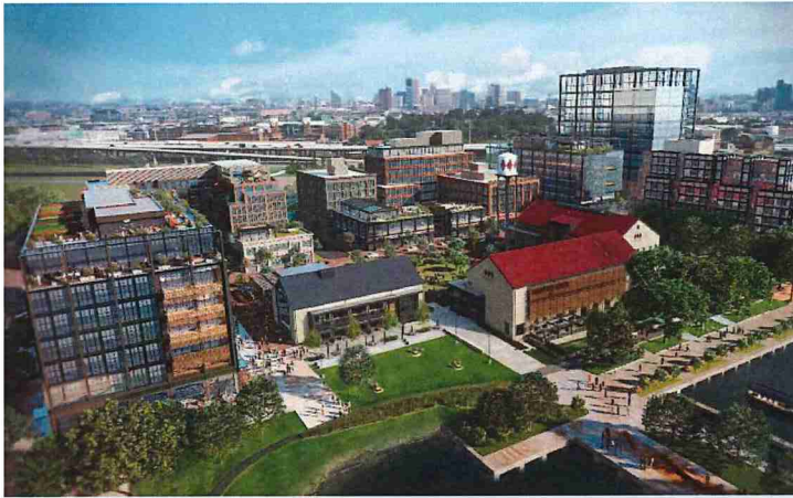
Port Covington in Baltimore will span 235 acres and feature 2.5 miles of waterfront. Weller Development will begin Chapter 1 of the $5.5 billion project this spring.
